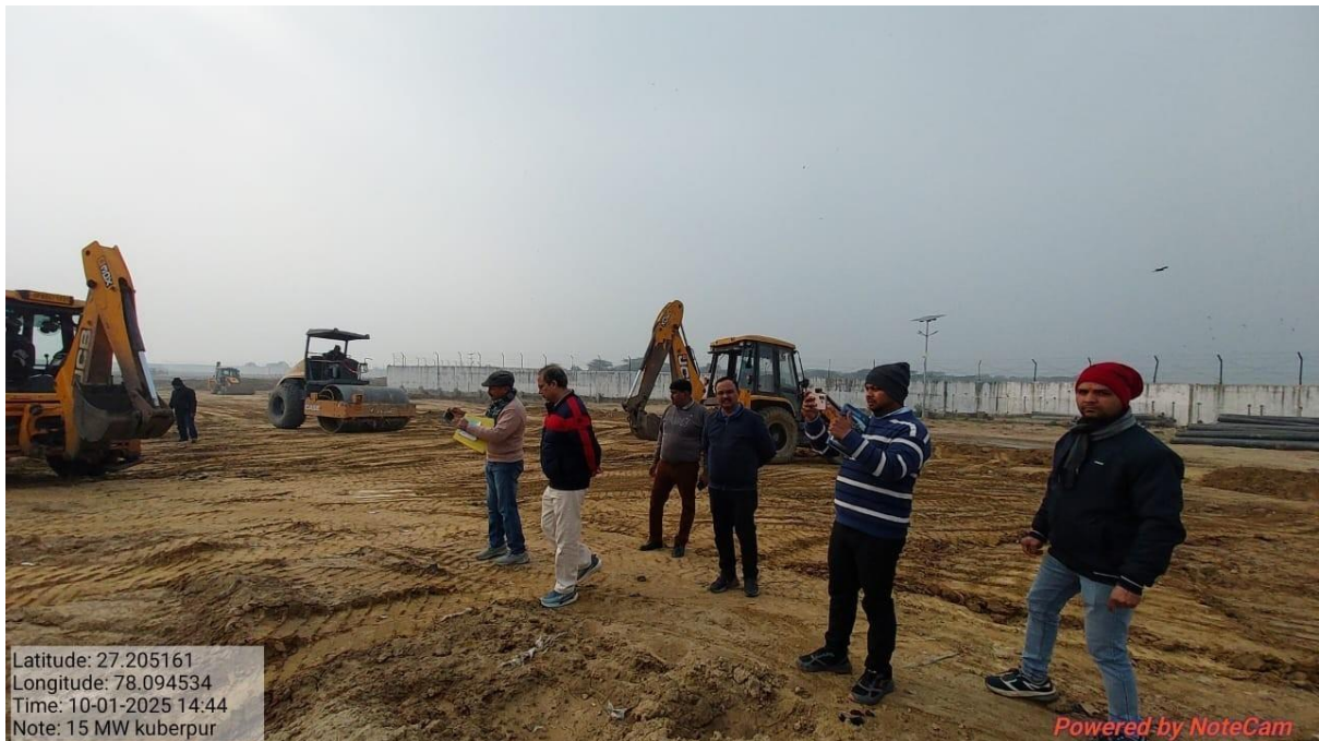
Pic-7- Land filling and levelling work in progress for WTE Plant
