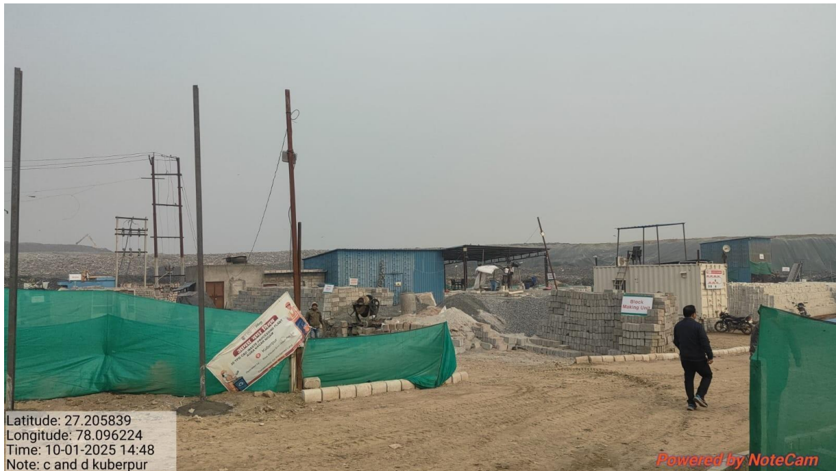
Pic-10- Functional C&D plant of Agra Nagra Nigam (20 TPD)
