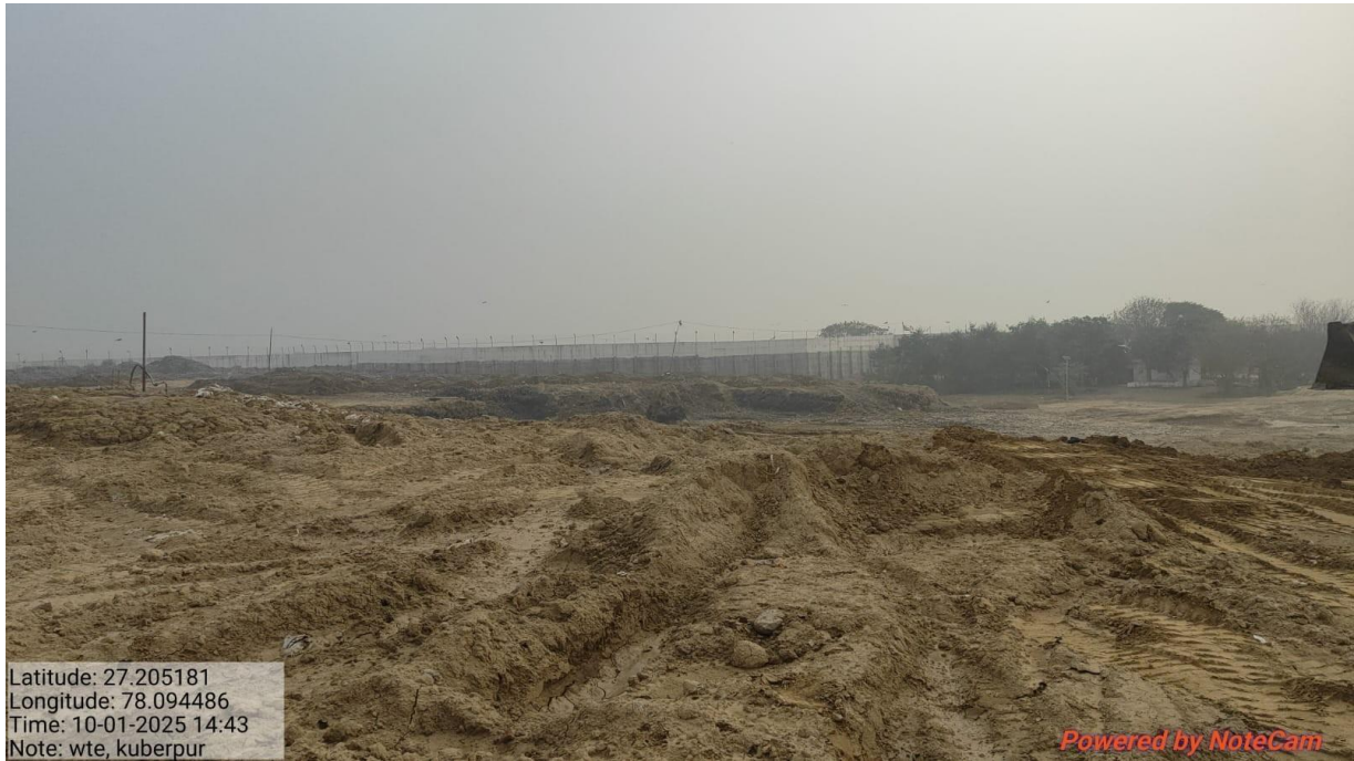
Pic-8- Land filling and levelling work in progress for WTE Plant
