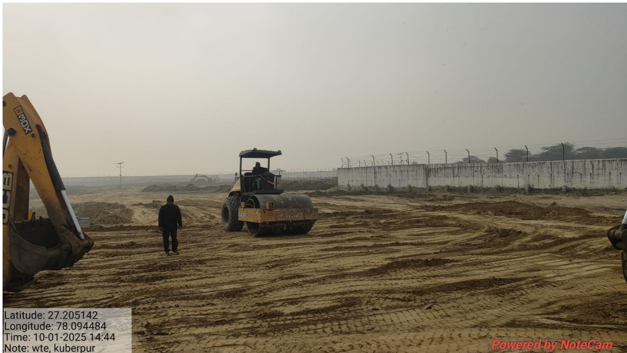
Pic-9- Land filling and levelling work in progress for WTE Plant
